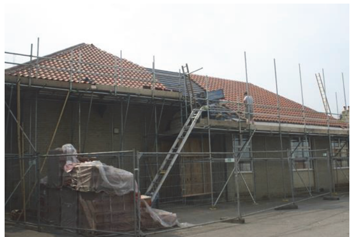
In 2006 a pitched roof was added to replace the 1965 flat roof.
